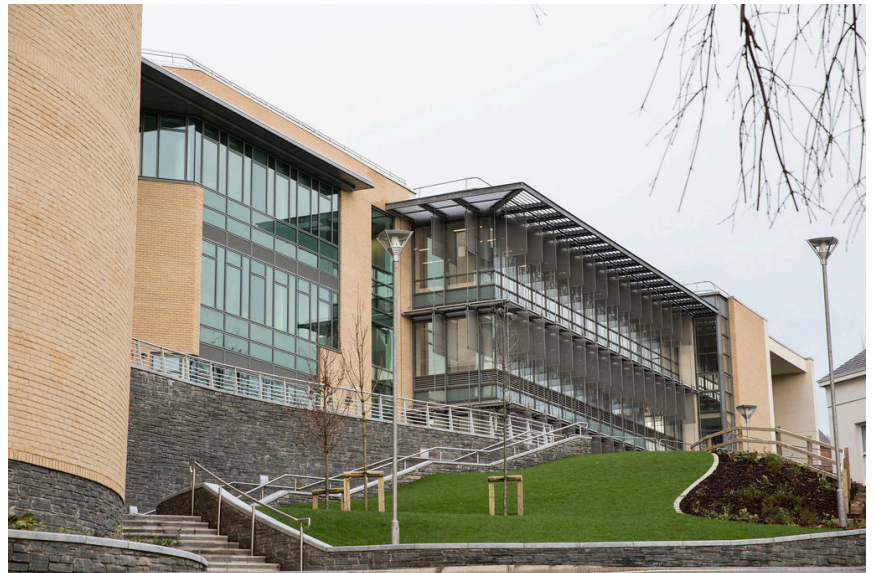
New facility at UU Magee Campus
